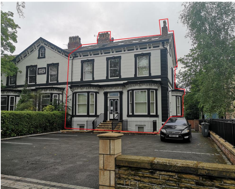
View of the front of 363 Wilmslow Road
