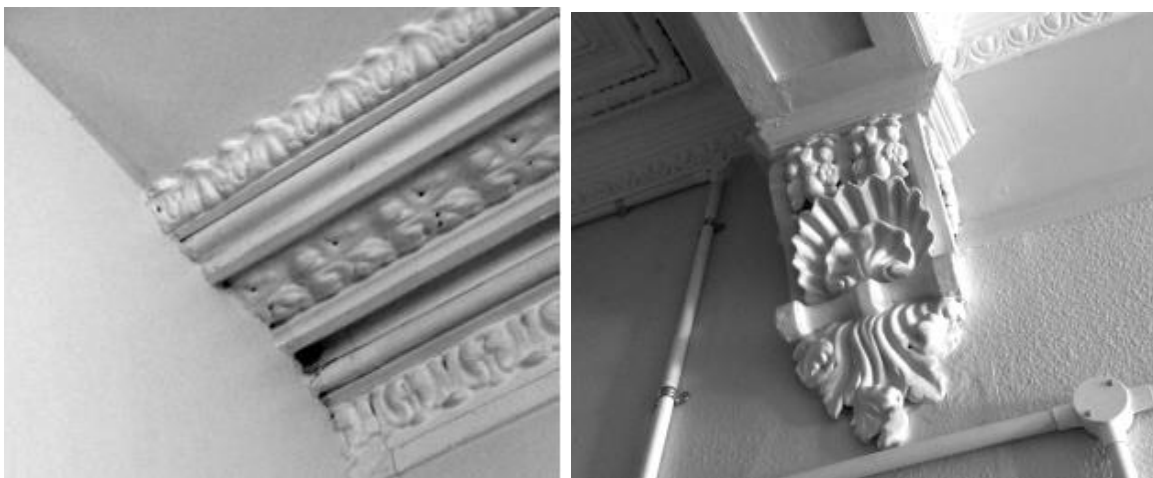
Cornice and Hallway console brackets to be reinstated
